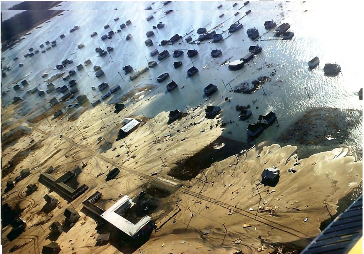
Aerial of damage and flooding from the Storm of 1962
