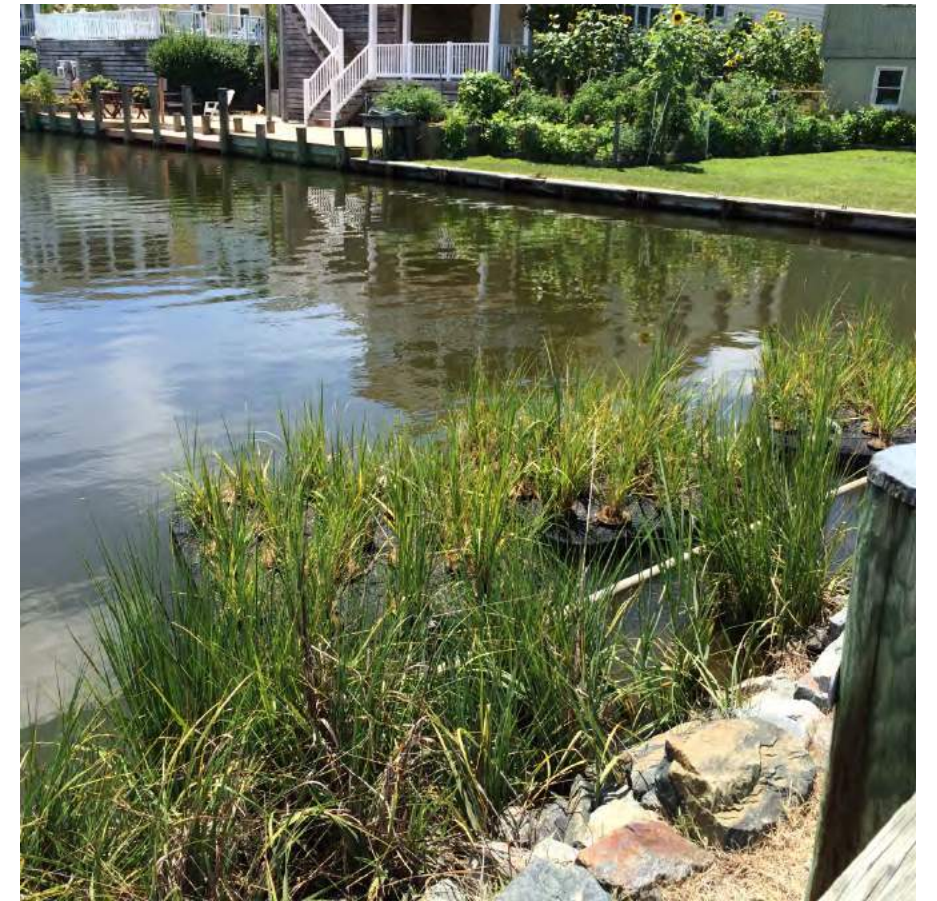
Floating wetlands installed on a canal to enhance water quality.
