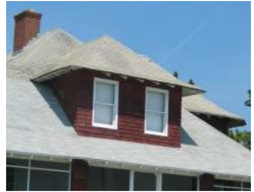
HIP ROOF WITH A HIP DORMER
