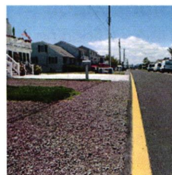
Figure 1: The Town of Fenwick Island installed an infiltration trench along Bayard Street to filter and store stormwater before draining to the canal.
