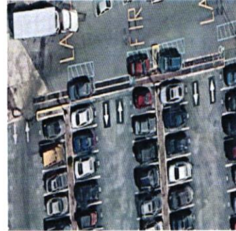
Figure 1: The above picture features an underground sand filter in a Newark, Delaware municipal parking lot.
