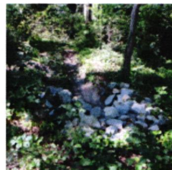
Figure 1: Rehoboth Art League Soil media, plants, and stones are used to filter stormwater before draining into a ditch system.
