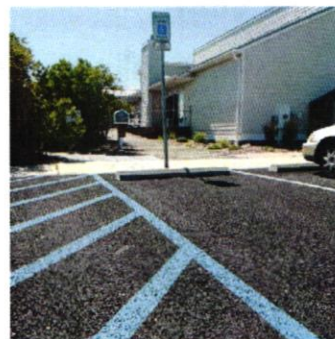
Figure 1: The Delaware CIB's main office located along the Indian River Bay. Their porous asphalt parking lot helps disperse water during high rain events.
