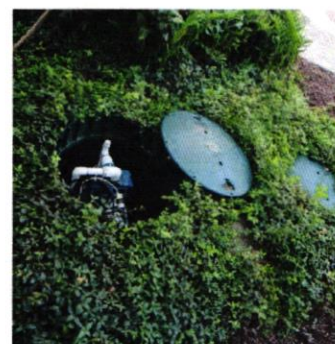
Figure 1: A resident of Lewes installed a 2,000-gallon cistern on site.
