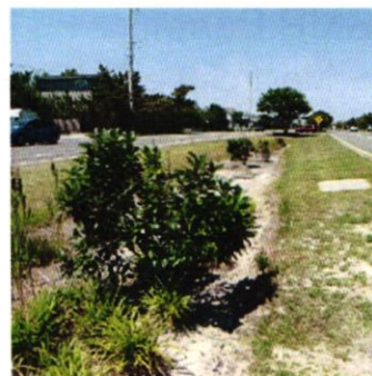
Figure 1: The Center for Inland Bays (CIB) worked with the Town of South Bethany to install bioswales in the medians along Coastal Highway (Route 1.)
