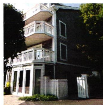
Figure 1: Canalfont Inn in Lewes has a system of drainage pipes that convey water from the roof to planted beds around the hotel.
