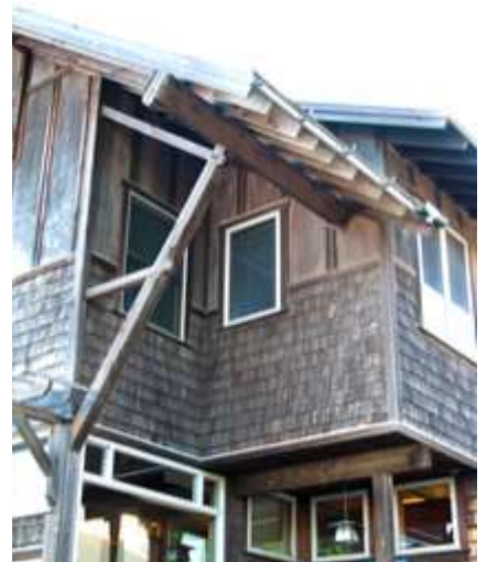
Exposed beams and rafters, combination board & batten and shingle siding
