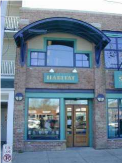
Flat roof with parapet and color accents. Arched canopy and recessed doorway provides desired relief.
