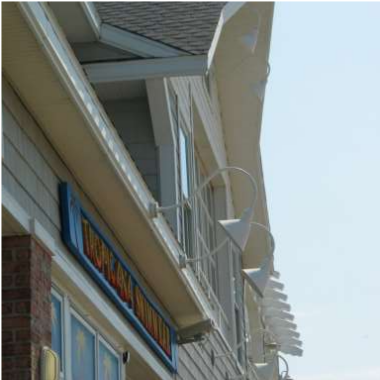
Shingle Style Details in light colors - Trim casing, composite shingles, trellis and rafter tails
