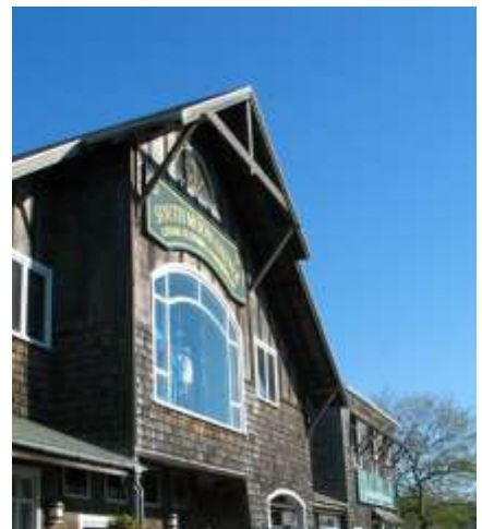
Gable truss and brackets in natural weathered wood
