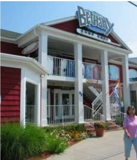
Example of porch as entry element, two-story columns and glazed-in porches as display windows.
