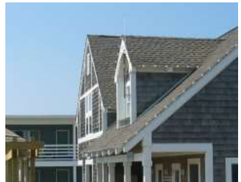
Large & small gable dormers with exposed rafter tails
