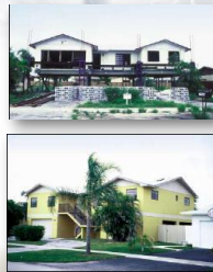
Top Picture: A house in Miami in the process of being elevated. Bottom Picture: That same house once completed. Taken from FEMA, Above the Flood, 2007
