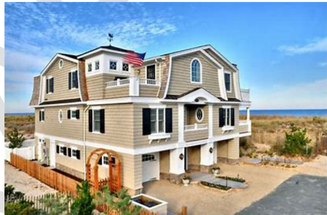
Newer home elevated on pilings
