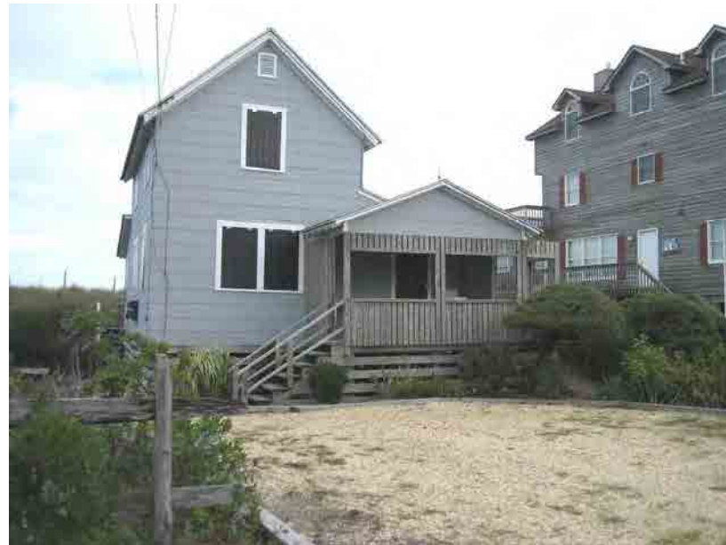
An original cottage.
