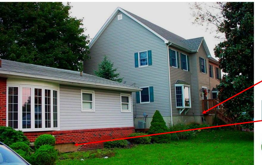
Lowest floor was built 1.5 feet above BFE - no damage
