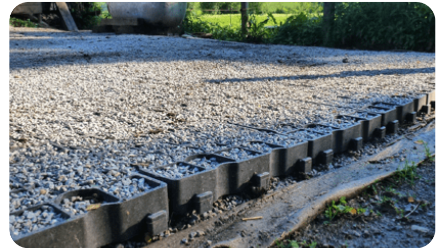
Stabilized Infiltration Trench
