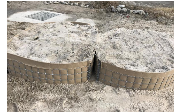
Sand-Filled HESCO Barriers to Reinforce Existing Bulkheads
