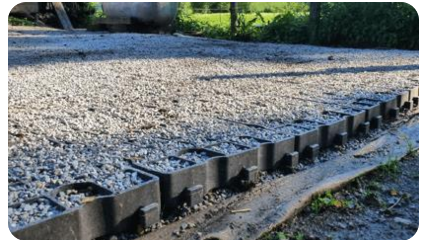
Stabilized Infiltration Trench
