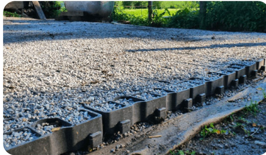
Stabilized Infiltration Trench
